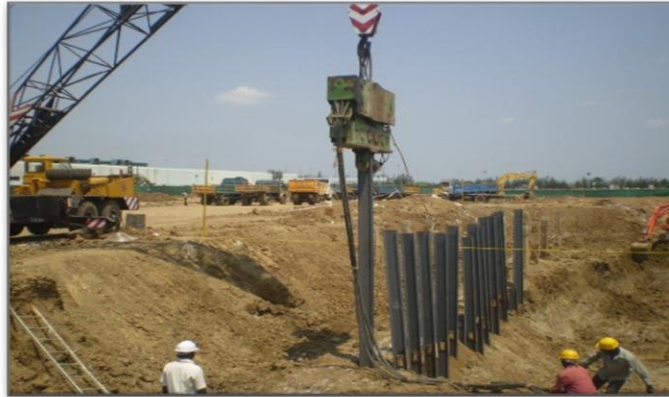
✓ Vibrant Hammer to Erect Shoring
